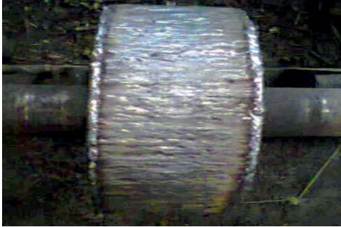
Crane Wheel Welding
