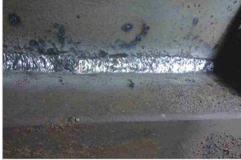
Arc Furnace Shell Crack Repair
